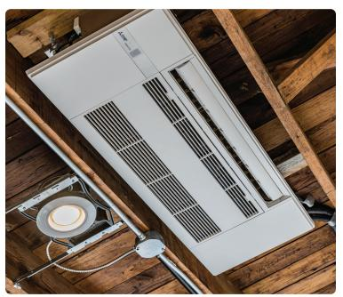
The EZ FIT® Ceiling-recessed Indoor Unit is designed to fit between standard ceiling joists, creating a flush appearance that is attractive to homeowners familiar with the sight of conventional vents. High/low ceiling airflow settings and automatic vane control provide personalized comfort, and the ability to fully service the unit from the bottom simplifies the maintenance process.
